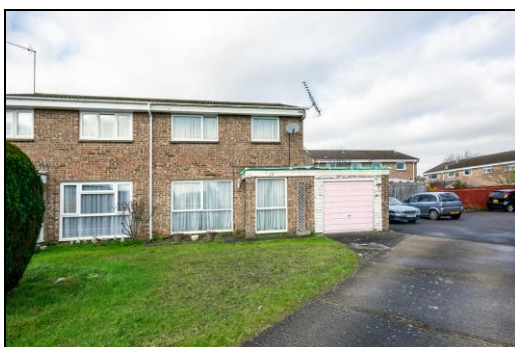
Front & Parking Area Access
